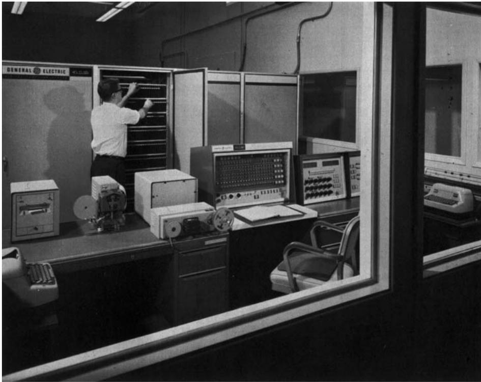
2 General Electric (GE) 412 computer was mainstay of hot and cold strip mill computer control worldwide during early 1960s: courtesy K. Morgan
