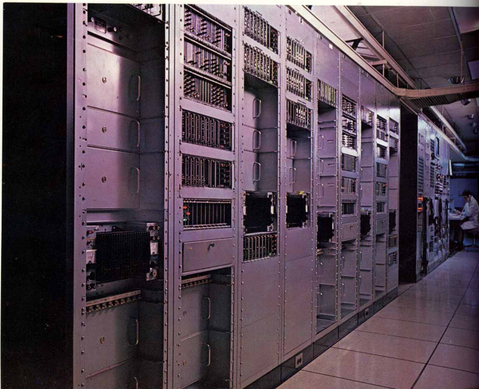
LONG VIEW OF VIDEO SWITCHING SYSTEMS looms large at the opposite end of OCR. Five TS-40 systems are housed here—assignment, Studio A, Studio B, master control, and house monitoring.
