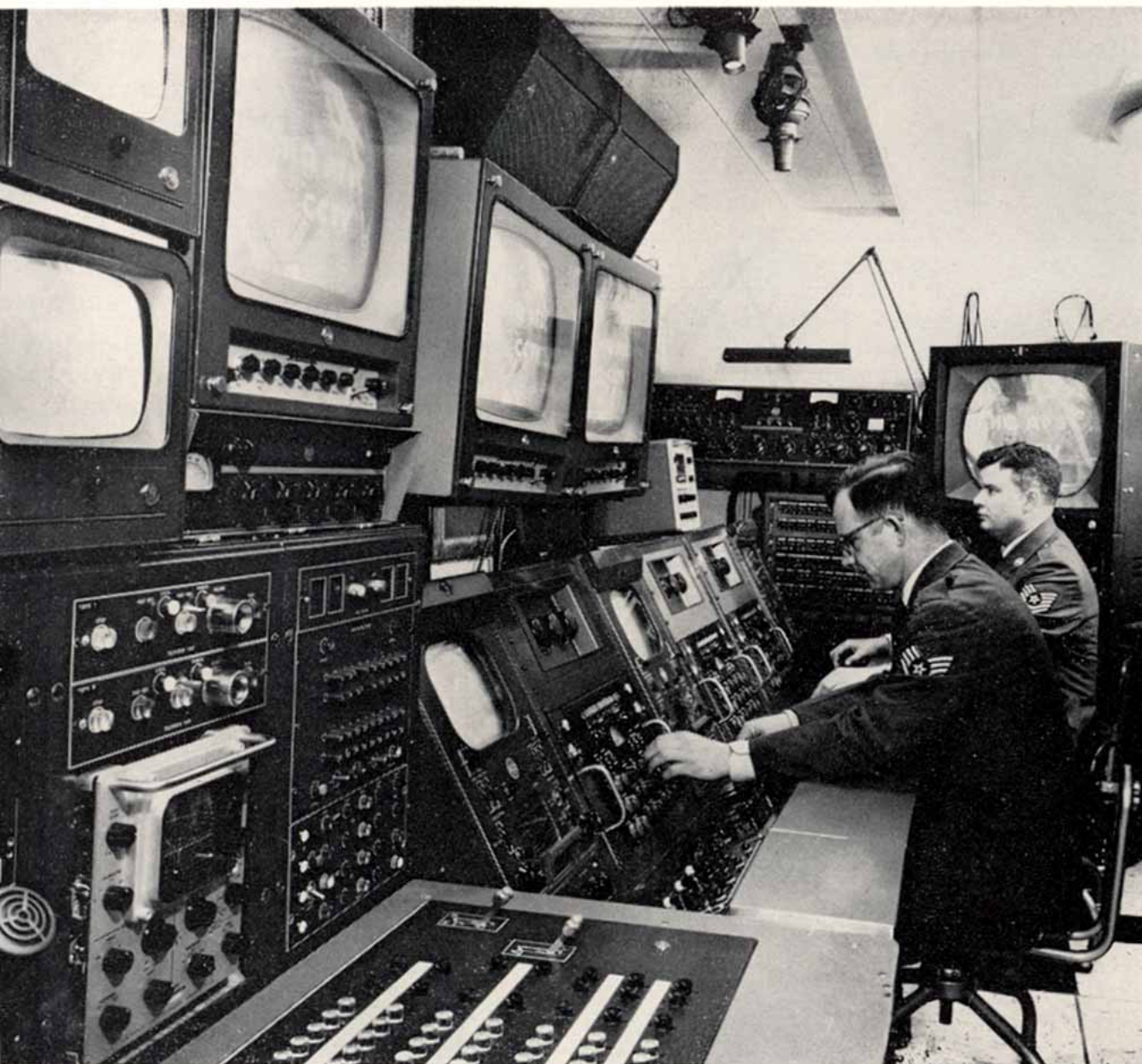
FIG. 10. Control room at Andrews for switching and control of color film and color studio cameras, and audio.
