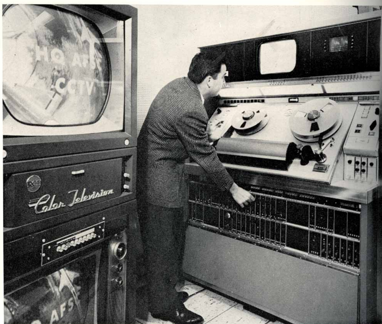
FIG. 16. Equipment complement at Andrews includes transistorized TV Tape Recorder, Type TR-22, for producing color briefings.
